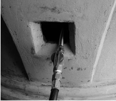
Figure 2C – Ball Valve Positioning
