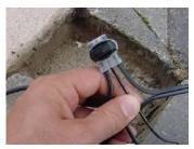
making sure that is it pushed all the way to the back. Finally take the black wire from a light and place it in the center hole, pushing it to the back of the connector. The connector should have 3 wires in it.
